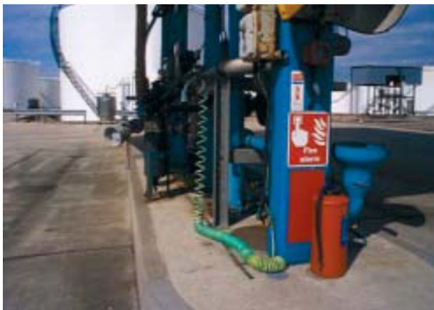
Figure 2. Typical bottom loading stand with provision for making earth connection to a tanker truck
