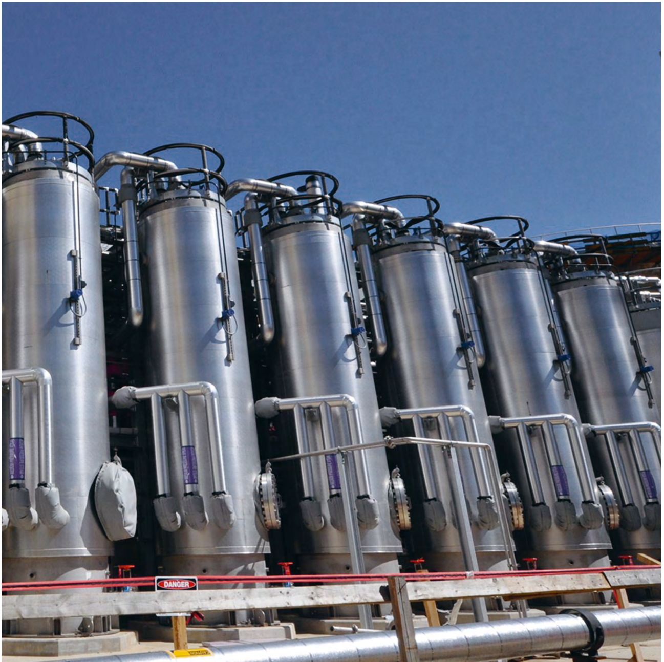
The world's largest Cambi plant for the production of biogas from sludge and waste, Washington DC. Photo: www.cambi.com
